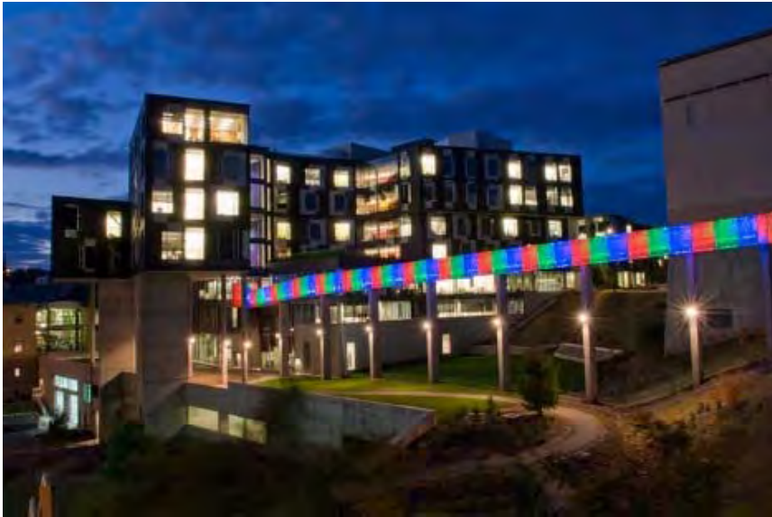
Pausch Bridge and The Gates Center at CMU
