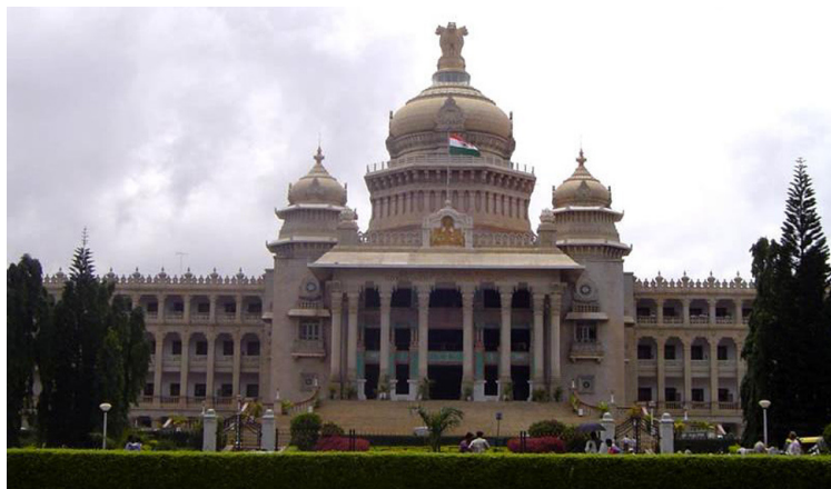
Vidhana Soudha, the stately building in the 'Neo-Dravidian' style, is located on Dr. Ambedkar Veedi road at the northern end of Cubbon Park. It houses the Secretariat, the State legislature and several other government offices in Karnataka.
